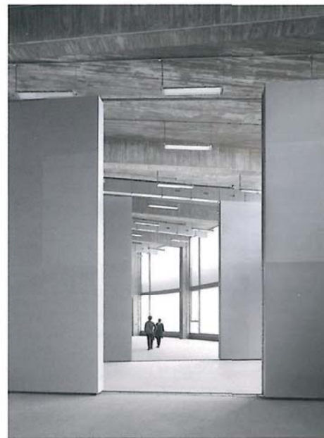
A continuous band distributes workshops and classrooms using a flexible organization that makes use of a modular structure of mobile dividing walls.
